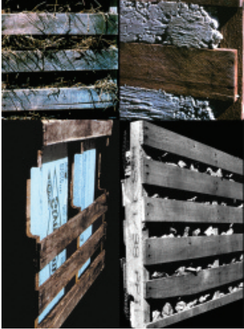
Above and below: During a crisis situation, pallet houses provide rudimentary shelter. Over time, inhabitants can transform them into permanent structures by filling in the gaps with whatever materials are available locally.
